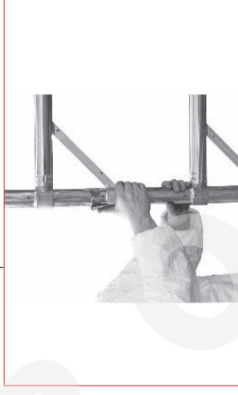
4 Klik in diagonal braces, starting at the bottom rung. Braces should be added in a continuous pattern. When fitting a full intermediate work platform it is permissible to interrupt the continuous pattern.
