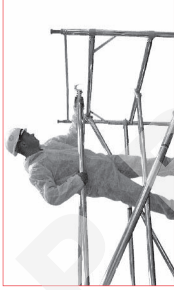
7 Fit four handrail braces, two on outside and two on mid rung of frame as shown, on lower levels these may not be required.
