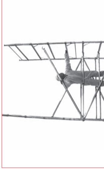
10 Klik in diagonal braces to continue in a regular pattern. Double width towers always have diagonal braces either side of the tower opposing each other as illustrated.
