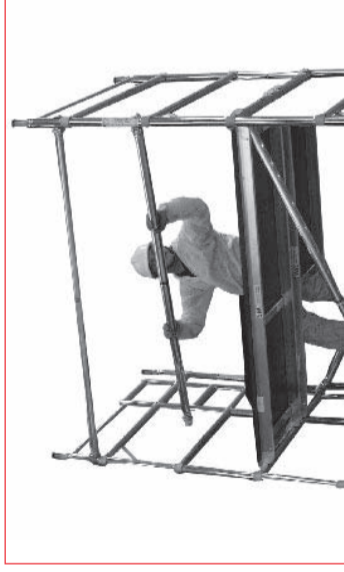
17 From the sitting position through the trapdoor (3T), fit four handrail braces to vertical member of frames.
