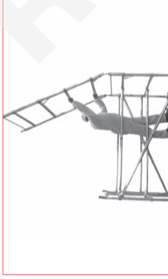
8 To add further frames, stand on platform ensuring the ladder frames are in line.
