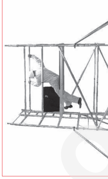
13 From the sitting position through the trapdoor (3T), fit four handrail braces, two on the outside and two on the inside as shown.
