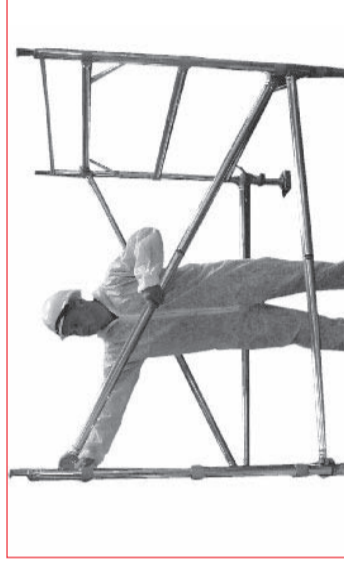
4 Klik in diagonal braces, starting at the bottom rung. Braces should be added in a continuous pattern. When fitting a full intermediate work platform it is permissible to interrupt the continuous pattern.
