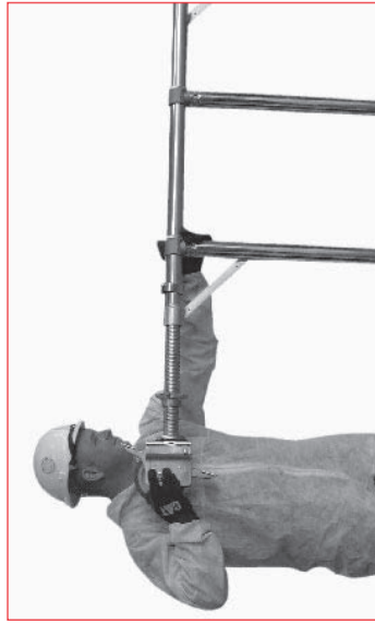
1 Insert two adjustable legs and castors into frame.
