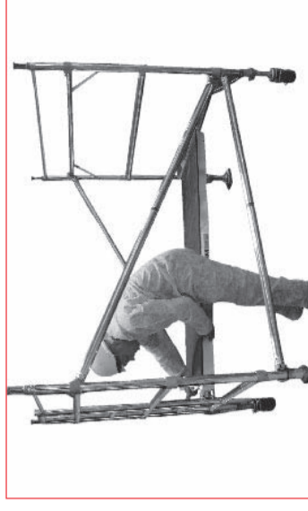
5 Fit plain platform on appropriate rung of frame. See lower kit guide for illustration. This will indicate which rung to fit trapdoor platform depending on final lower height.
