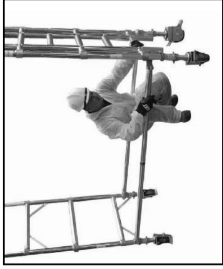
2 Fit in 2 horizontal braces to the vertical member of the frames, as low as possible, below the 1st rung. All horizontal braces fit on from inside the tower facing out.
