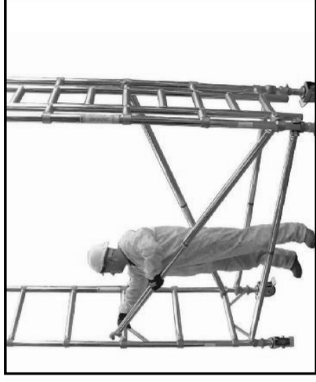
4 Facing the plain frame fit 1 diagonal to the bottom rung as close to the right hand frame vertical as possible. Facing the ladder frame fit 1 diagonal to the bottom rung as close to the ladder as possible.
